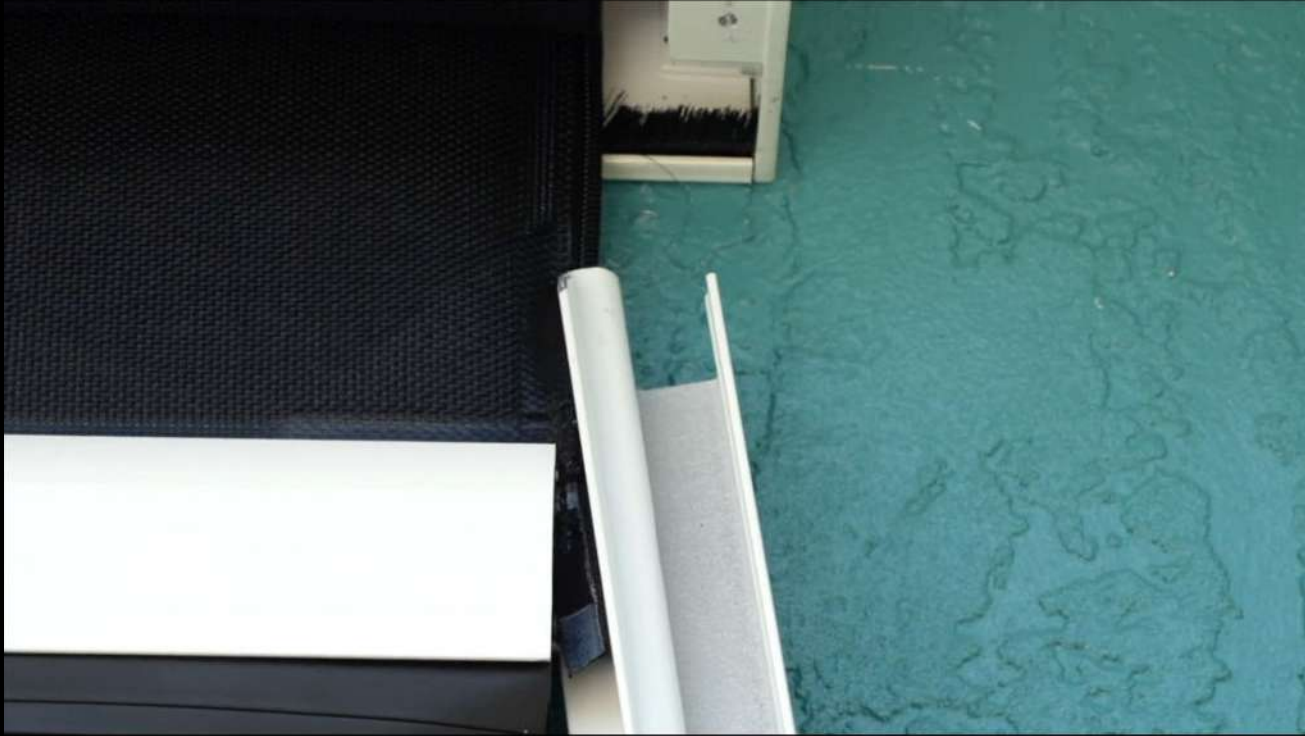
Angle tracks to ensure screen guide enters top funnel
