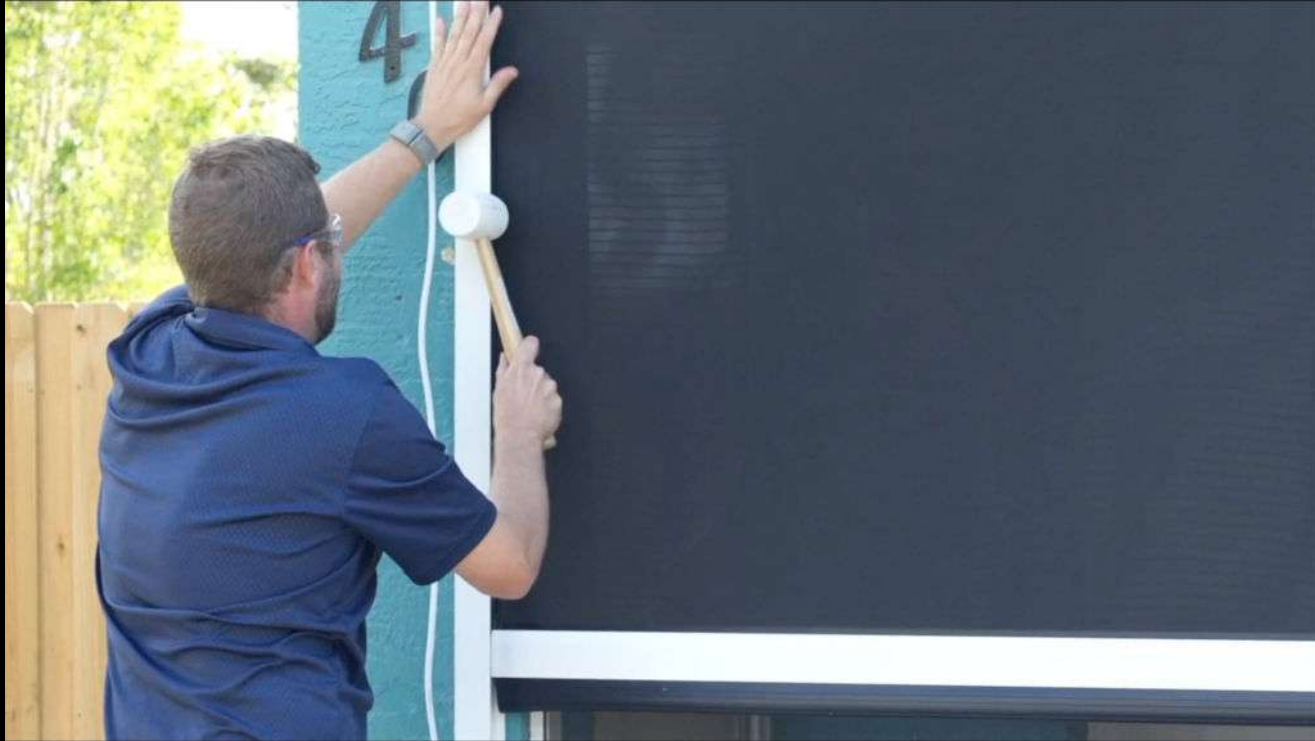
Attach track covers using rubber mallet
