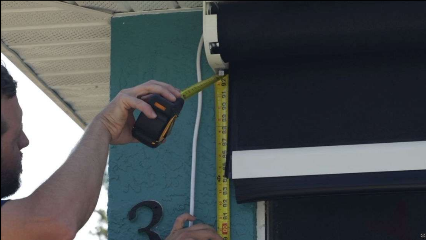
Measuring tacks before cutting tracks
